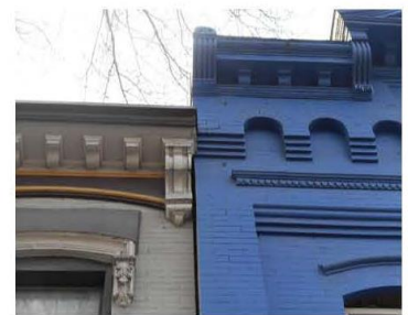
BUILDING @ PROPERTY LINE
